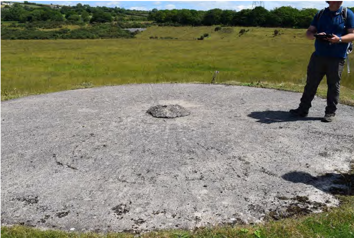
Photo 7: Shows one of the two capped mine shafts at the top of the slope on the southwest of the site
