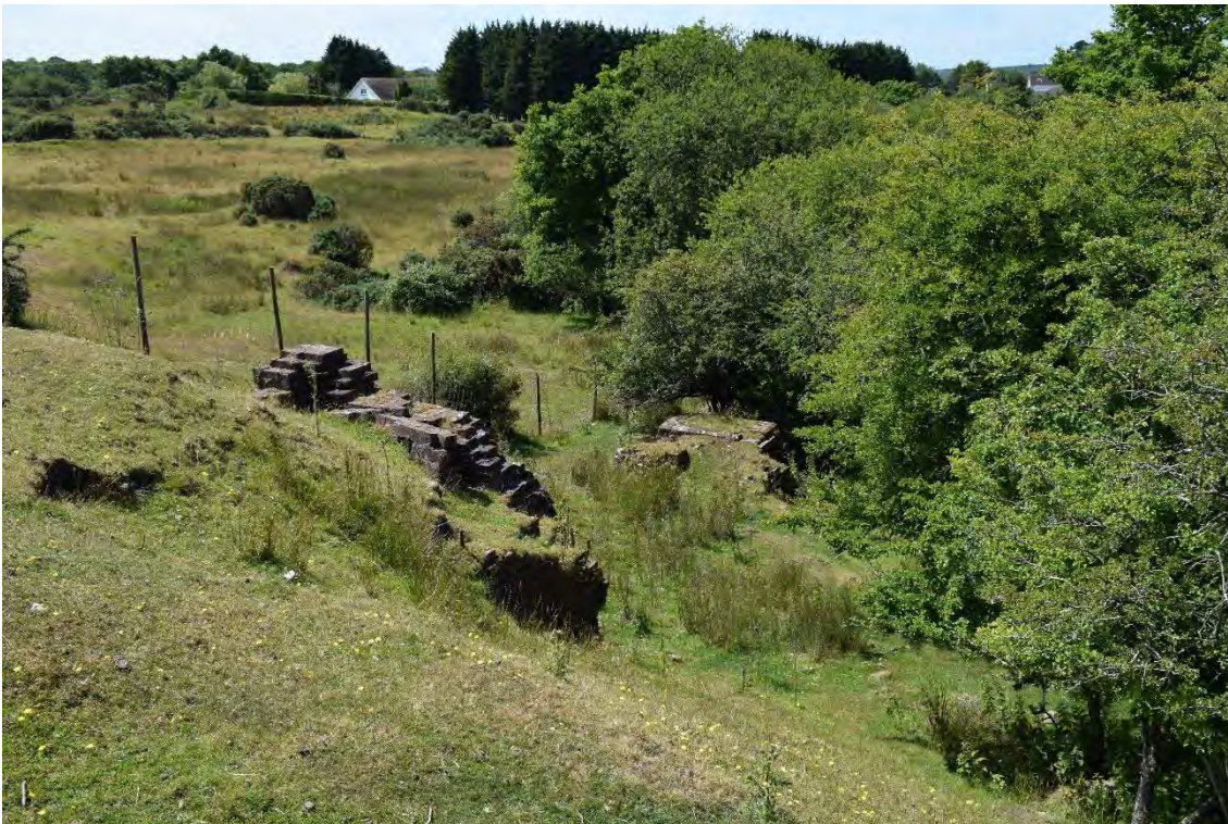
Photo 8: Shows redundant and relic brick structures in the southwest corner of the site.
